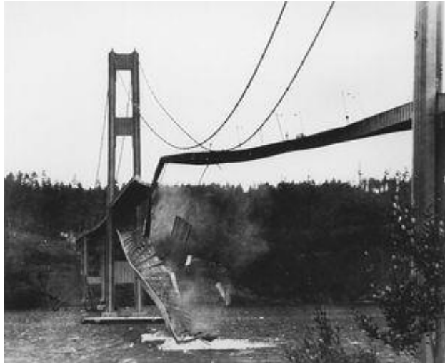
Tacoma Narrows Bridge Collapse of the Tacoma Narrows Bridge, Washington state,
